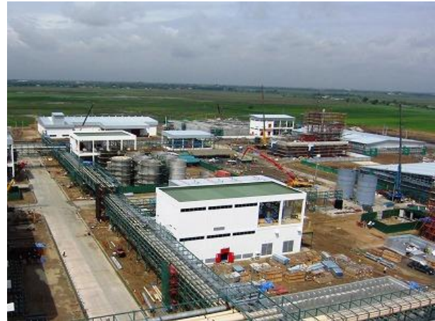
Facilities under construction
