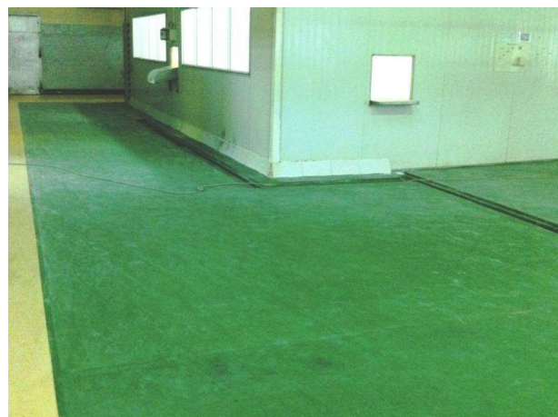
New floor surface
