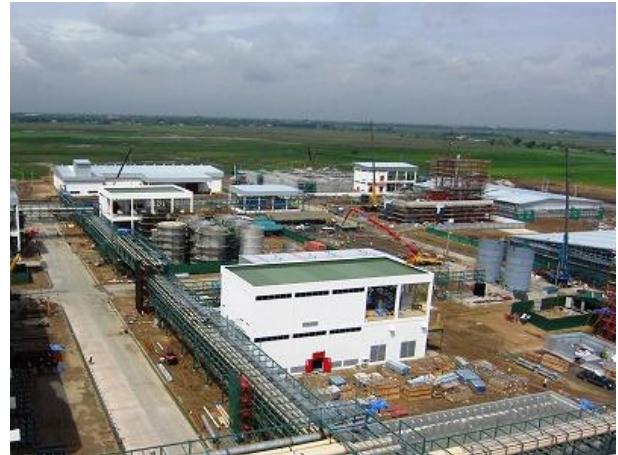
Facilities under construction
